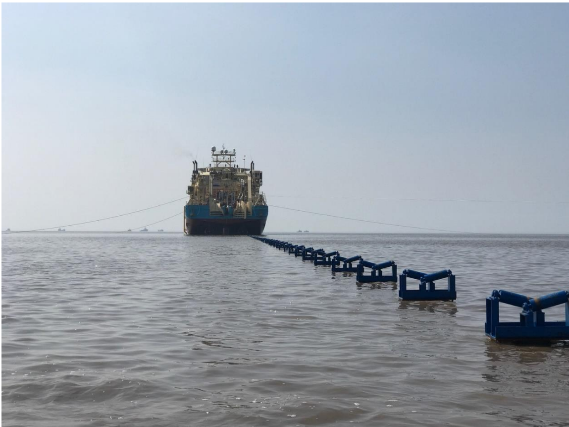
Plate 4.1 Example CLB in position using a mooring system with cable rollers in the foreground (Walney Extension Offshore Wind Farm)
